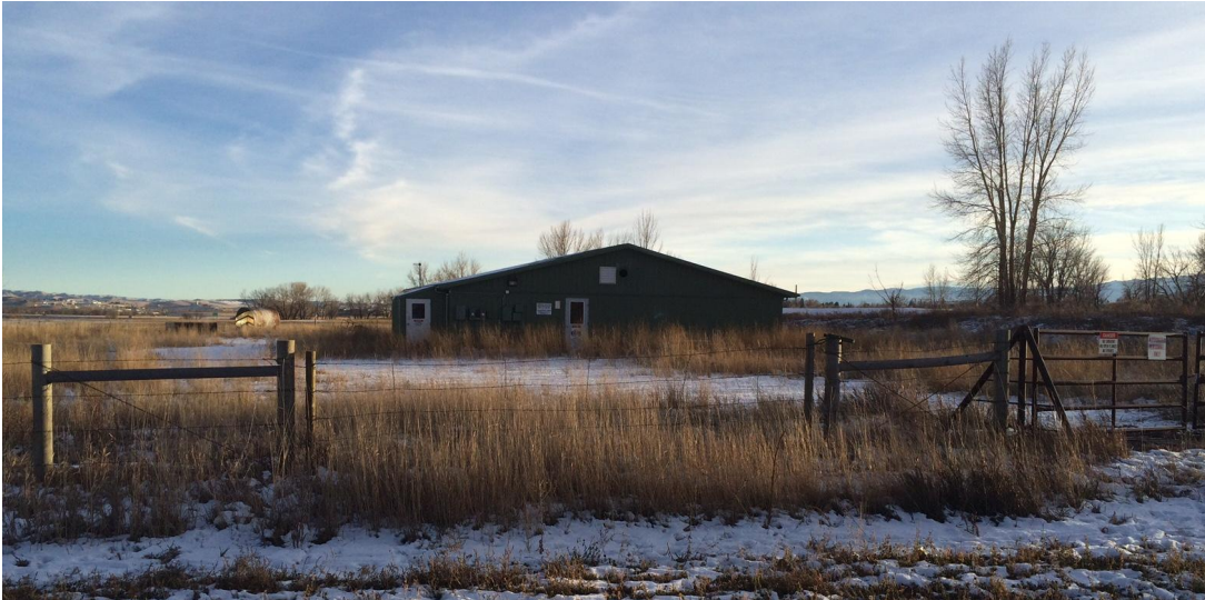
Figure 3.2. Un-reclaimed compressor station, Sheridan County, WY (Source: author)
